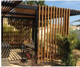
Timber pergola with in-filled roof/walls
