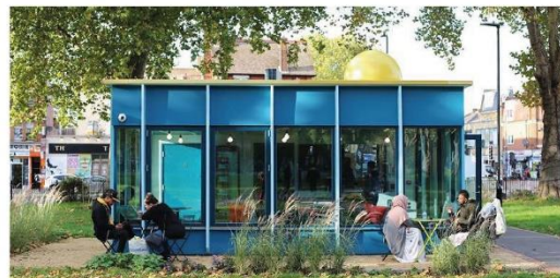
Natural surveillance from the active frontages of the community hub building located close to sports and play provision
