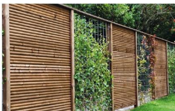
Boundary to the community garden incorporating planting
